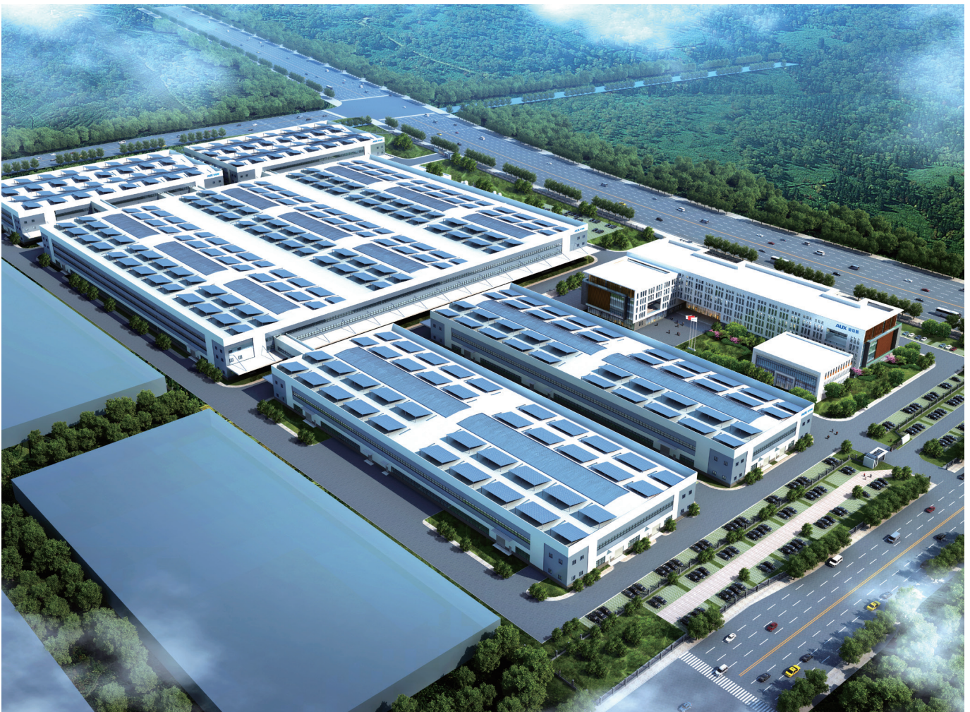
Smart Factory · Ningbo
