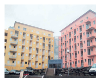
Vannia Park University Dormitory FRANCE
